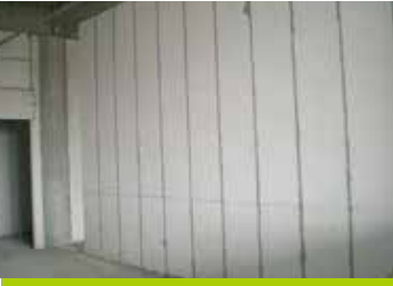
Initial Installation Completed
