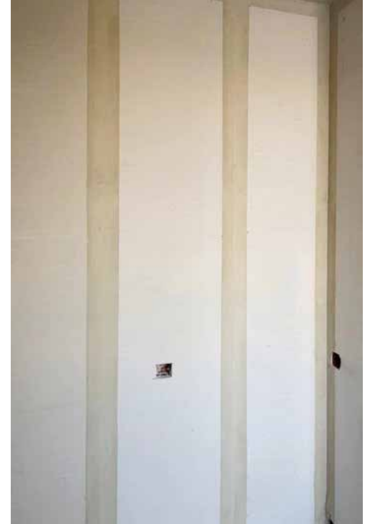
Finished Installation of AAC Integrated Conduit Panels
