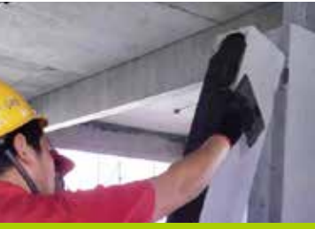
Apply Mortar (Adhesive)
