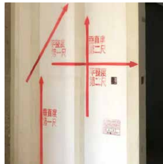
AAC Integrated Conduit Panel Installation Site
