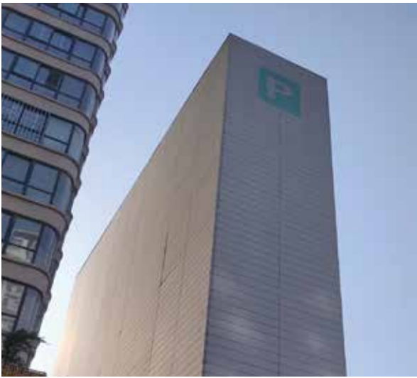
AAC Exterior Wall Panels - Fully Completed
