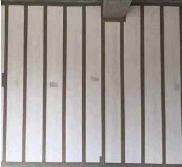
AAC Interior Wall Panels - Full-Wall Mesh Application
