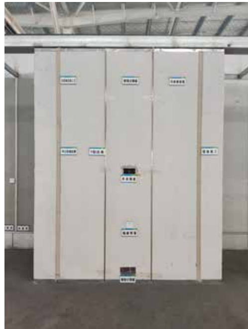
Finished Installation of Cavity Wall
