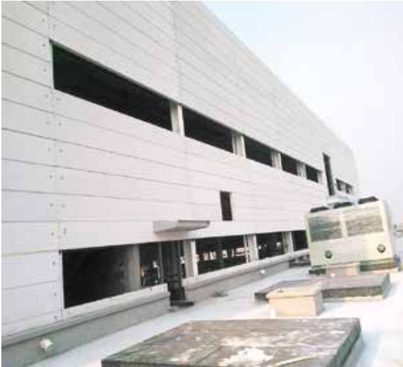
AAC Exterior Wall Panels - Fully Completed
