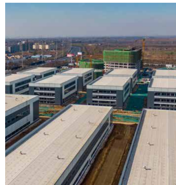
Luoyang Zhongyuan Environmental Protection Park Application: Fortera high-precision AAC blocks.
