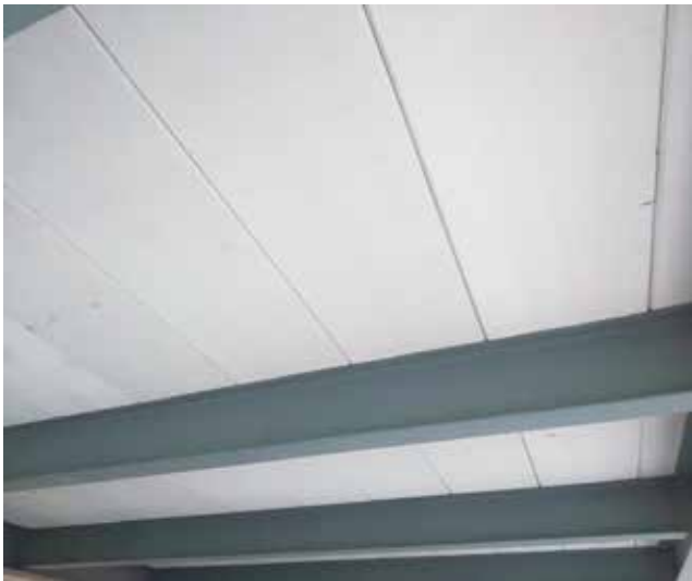
AAC Floor Initial Installation Effect
