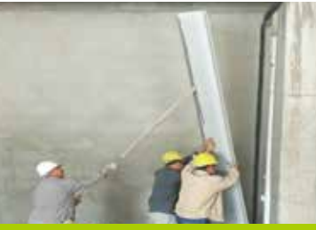
Erect the Panel
