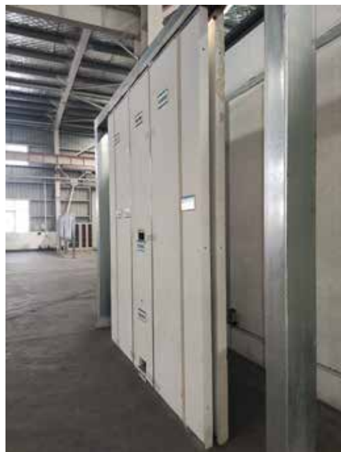
Finished Installation of Cavity Wall
