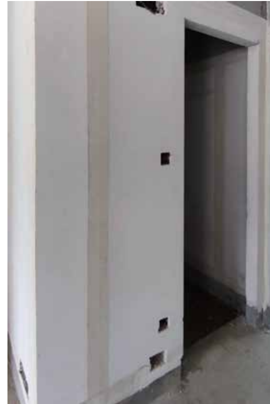
AAC Integrated Conduit Panel Installation Site
