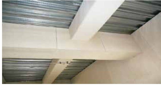
AAC Fireproof Panel Beam Initial Installation Effect
