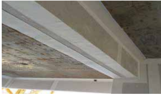
AAC Fireproof Panel Beam Initial Installation Effect
