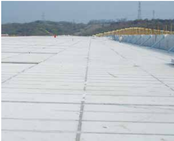
AAC roof panel initial installation effect
