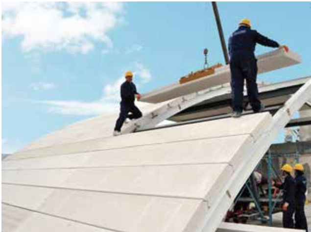
AAC roof panel installation process
