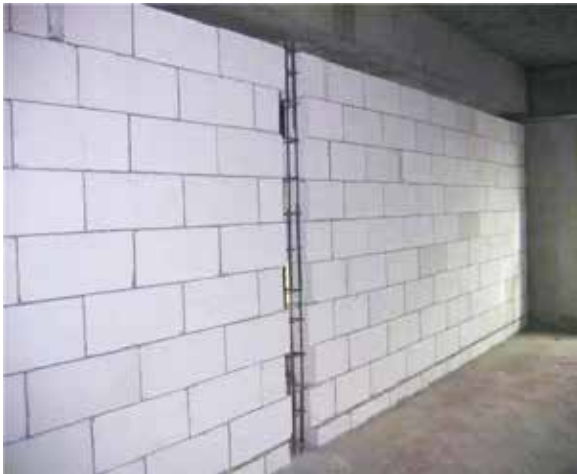
AAC Block Initial Installation Effect
