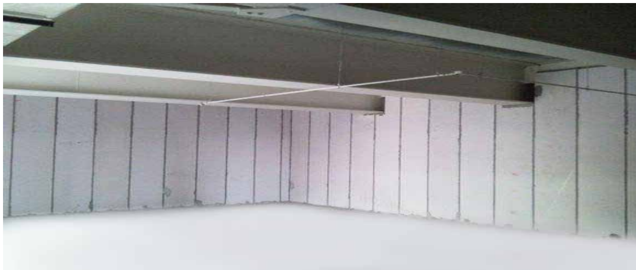
AAC Fireproof Panel Beam Initial Installation Effect
