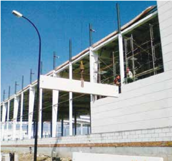
AAC Exterior Wall Panels - Initial Installation
