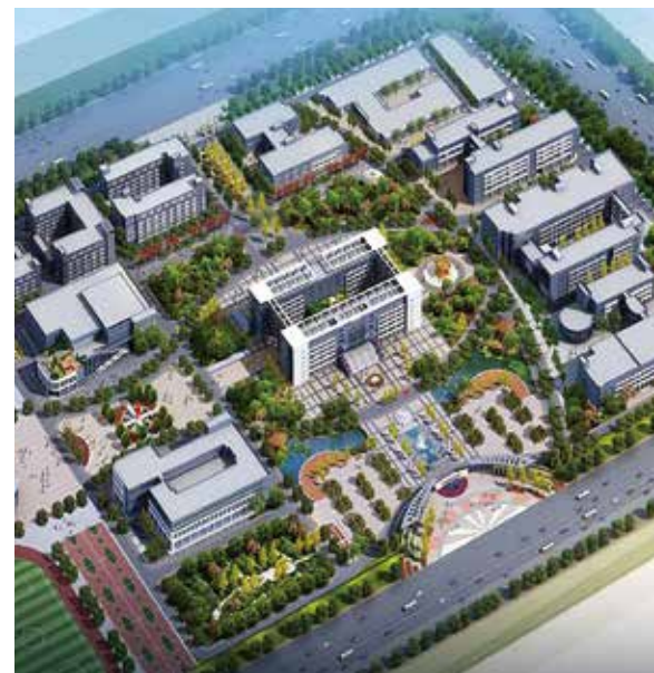
Jiaozuo Vocational & Technical College Area: 225,800 m 2 Application: Fortera AAC interior panels.
