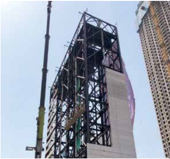
AAC Exterior Wall Panels - Initial Installation
