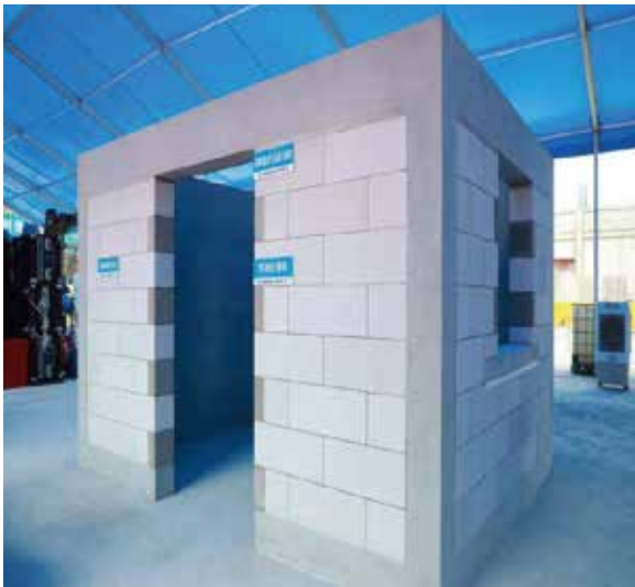
AAC Block Initial Installation Effect
