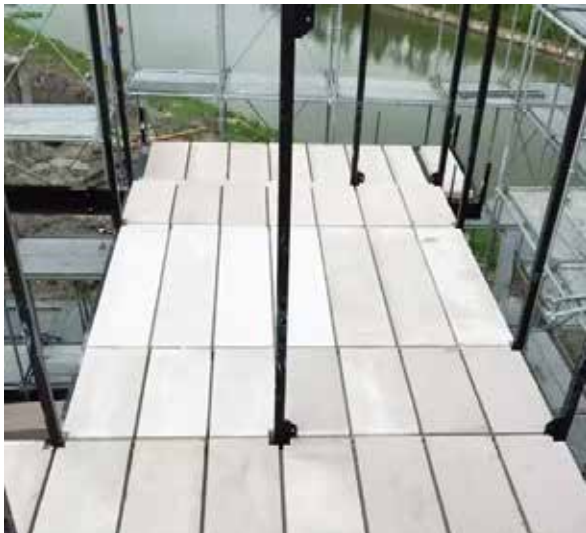
AAC Floor Installation Initial Effect From Above View
