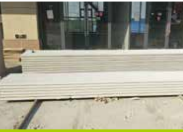
Deliver & Stack Panels on Site
