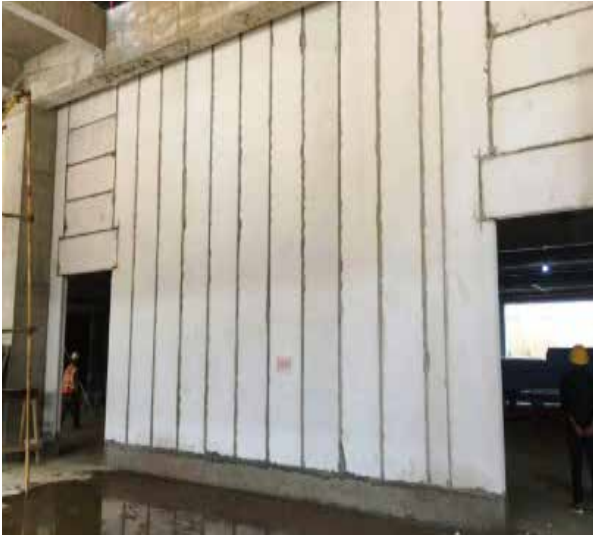
AAC Partition Panels - Initial Installation
