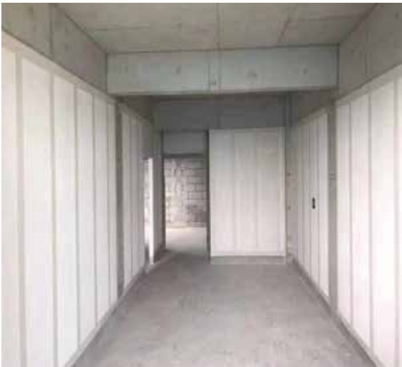
Residential AAC Interior Wall Panels - Initial Installation
