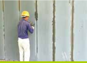
Joint Grouting
