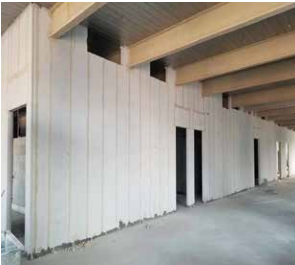
Factory AAC Interior Wall Panels - Initial Installation
